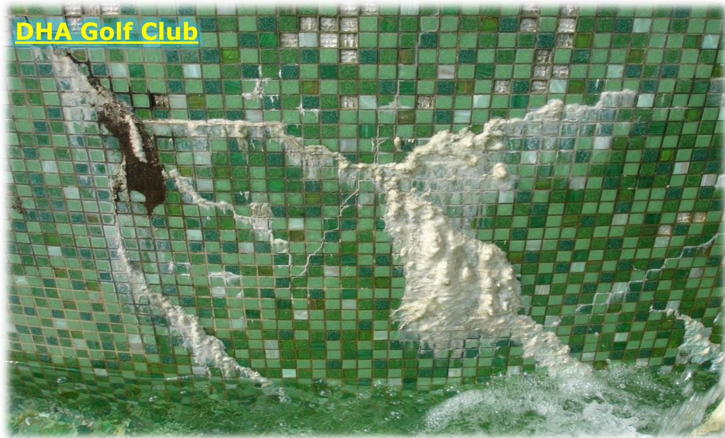
Close up of free lime accumulation
